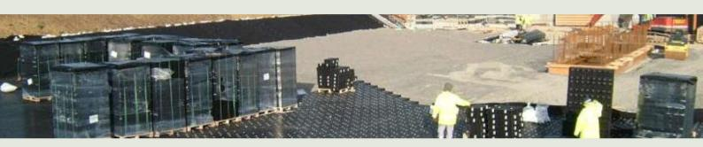
Fire training drills left a legacy of hydrocarbon and foam contam in the near surface soils. The Contract comprised the construction of an evaporation cell to retain and reuse precipitation falling on the site. The cell design was by Professor John Knapton and comprised a permeable paving system isolated from the surrounding ground capable of supporting repeated heavy vehicle loading.
