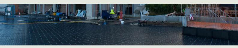
Multi-phase development by Durkan partnering with London and Regional Properties to provide apartments. Areas between the blocks included community space with recreational areas. SEL installed a Permavoid podium deck drainage system provided a very shallow (85mm) high strength, highly efficient drainage collection and attenuation system. The podium deck was c.7,600sq.m
