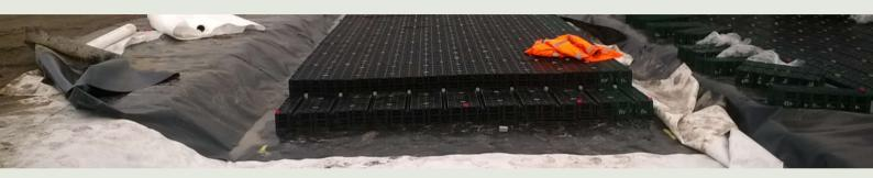
Due to the site being on Brownfield land, having a high water table and a shallow outfall, a shallow solution would negate the need for pumping stations and reduce the need for temporary works.
