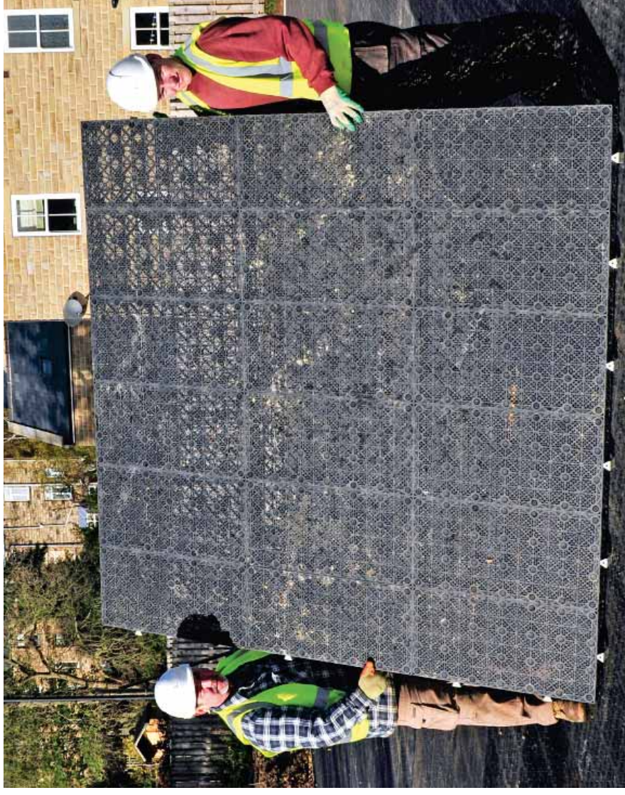
Permavoid assembled in a 2.124m x 2.124m panel
