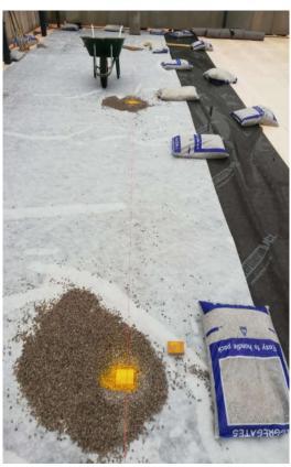
Protective geotextile is rolled out over the area.
