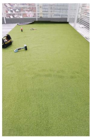
Rolls of synthetic grass are positioned in the correct location in line with the manufacturers roll-plan.
