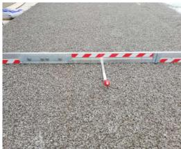
Gravel is deposited in bays and levelled by hand.
