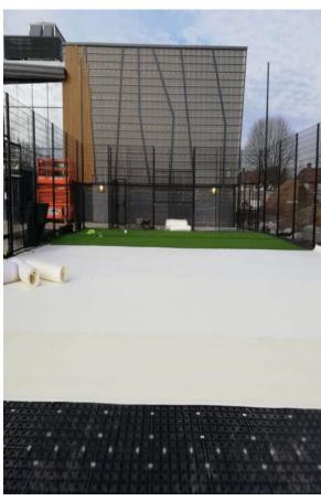
Rolls of pre-fabricated shockpad are rolled out over the area.
