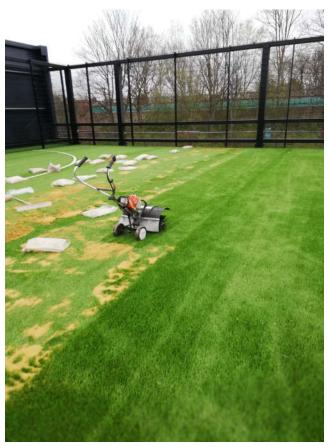
Silica sand infill is distributed over the synthetic grass in accordance with the grass manufacturers recommended spread rate.
