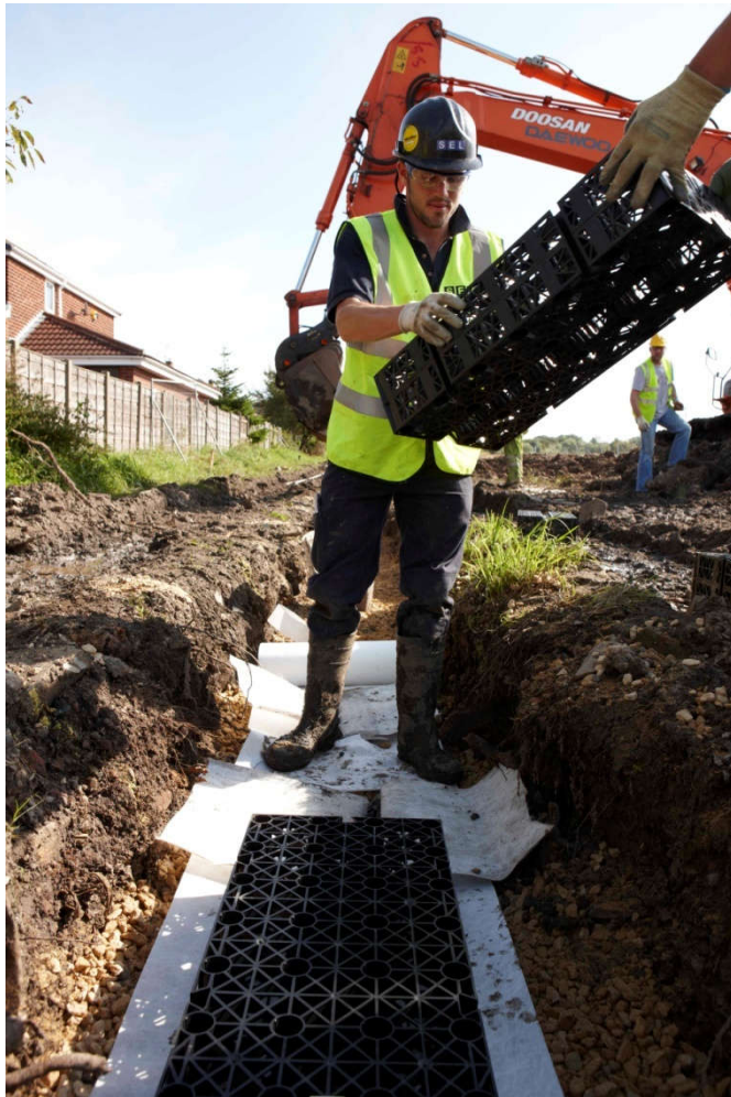
Lay geocellular duct
